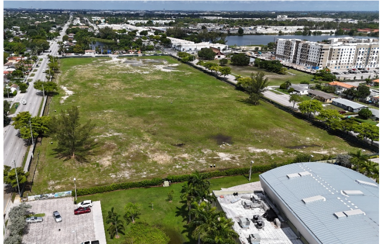
Project site facing west (Claude Pepper Park Joe Celestin Center can be seen in the bottom right foreground)
