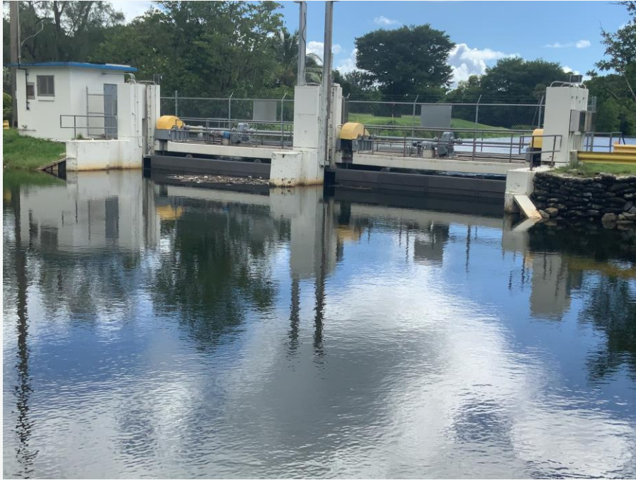
Photo: S-28 Spillway Structure on October 08, 2025 (Looking Downstream from Upstream)
