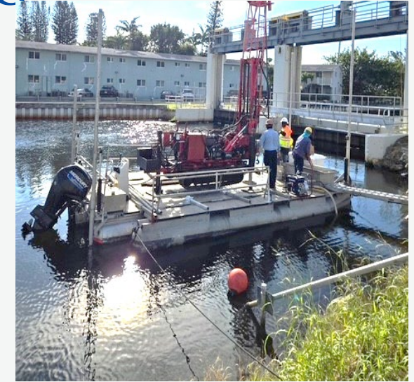
Geotechnical Investigation at S-27 Spillway
