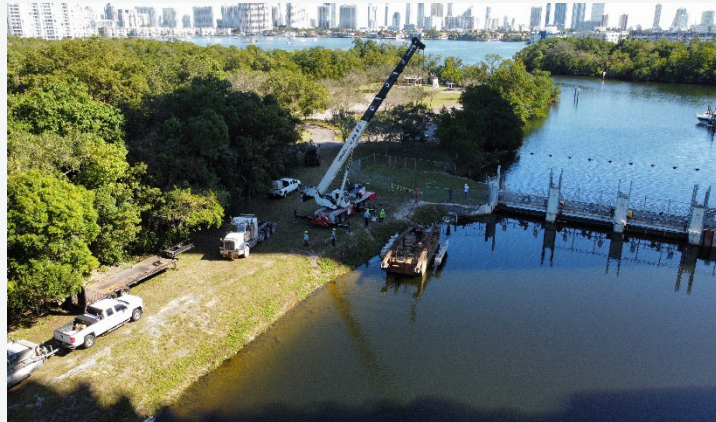
Geotechnical Investigation at S-29 Spillway
