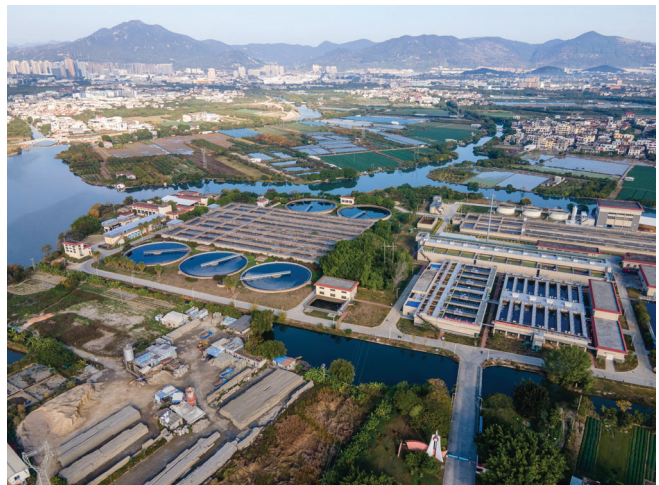
Reverse Osmosis Water Treatment
