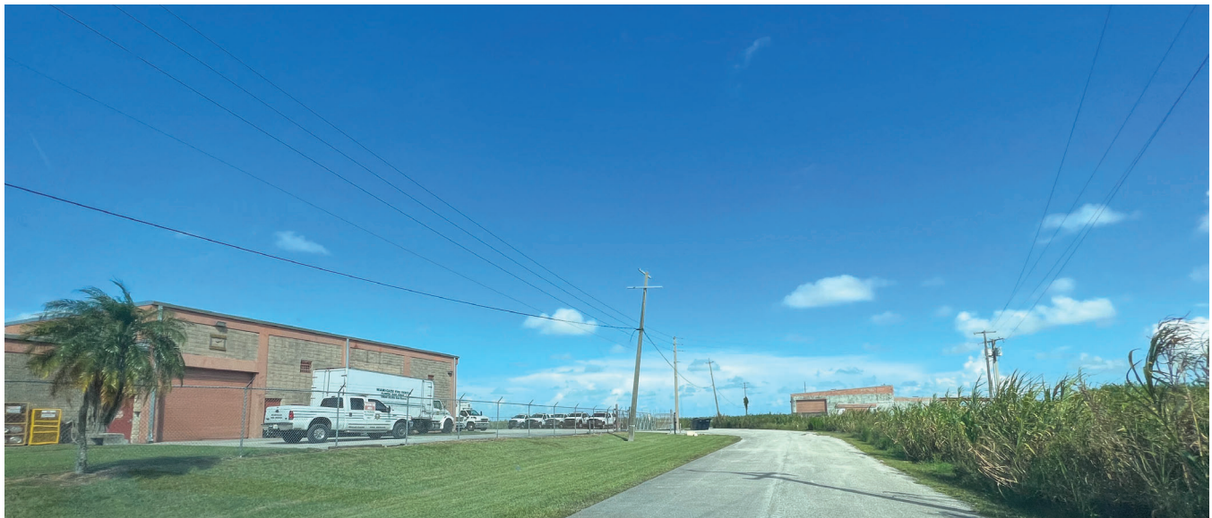
Power Infrastructure at HARB
