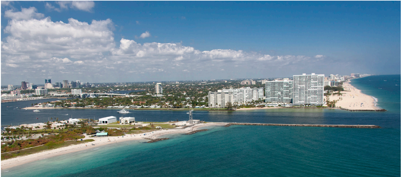
SFOM North Site at the Port Everglades Inlet
