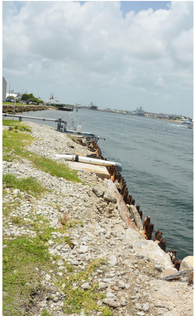
Eroded Seawall
