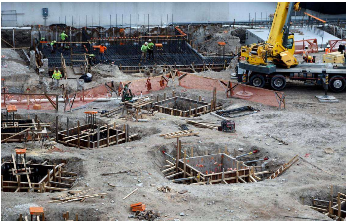
Construction on a $500 million multi-year project is underway at the Bal Harbour Shops in Bal Harbour, Florida, on Wednesday, January 10, 2024. Al Diaz adiaz@miamiherald.com
