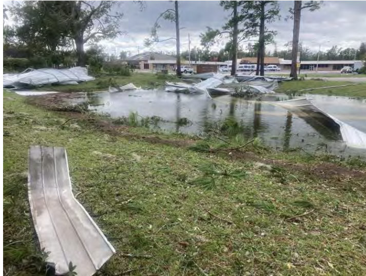
Taylor County sustained flooding and other widespread damage in Hurricane Idalia. Mike Exline
