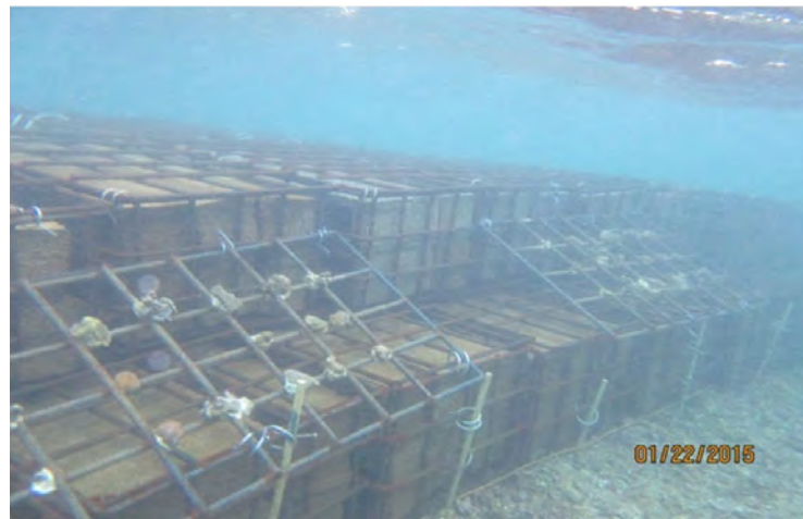
Figure 20. A hybrid CR4 structure installed in Grenada to reduce wave energy. Photo credit: TNC.
