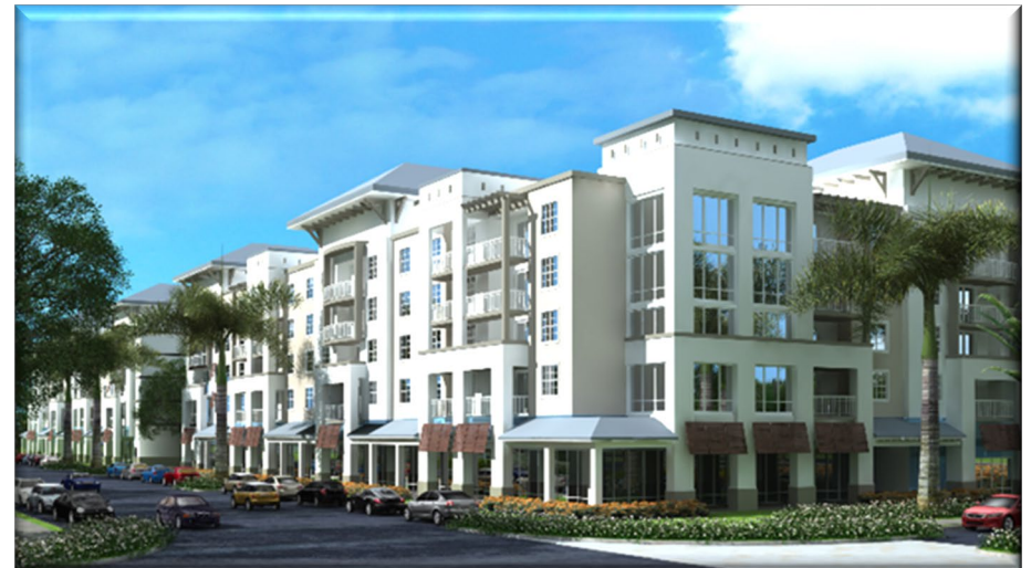
Liberty City Square Redevelopment Project, Miami-Dade County
