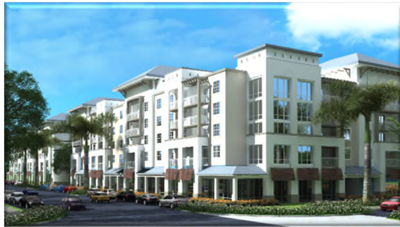
Liberty City Square Redevelopment Project, Miami-Dade County
