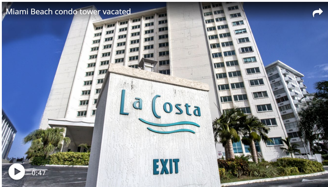
A Miami Beach condo tower, built in 1964, was vacated by city order and faces demolition and a developer buyout after failing for years to complete required repairs.
