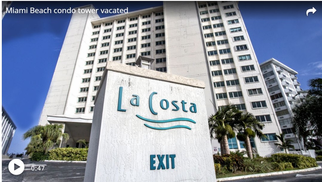
A Miami Beach condo tower, built in 1964, was vacated by city order and faces demolition and a developer buyout after failing for years to complete required repairs.
