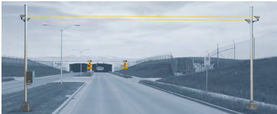
ROADWAY CCTV CAMERA AND TRAFFIC SENSOR (MDVS)
