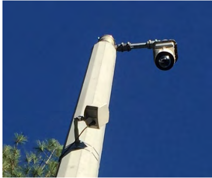
ROADWAY CCTV CAMERA AND TRAFFIC SENSOR (MDVS)
