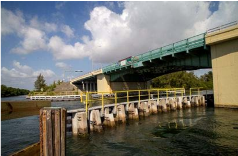
The Dania Beach Boulevard bridge. A study from Florida Atlantic University in 2012 found that the lowest-lying state road in Florida was Dania Beach Boulevard. (Pedro Portal/Miami Herald)
