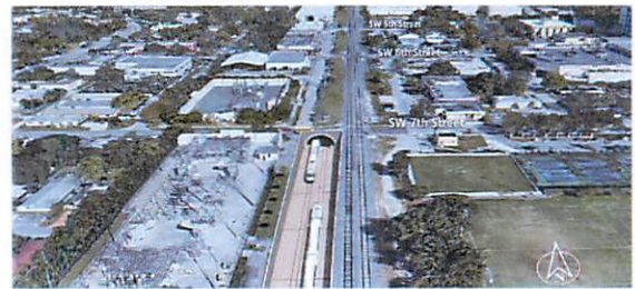
Tunnel beneath New River
