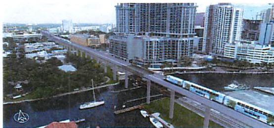
80-foot high-level fixed bridge
