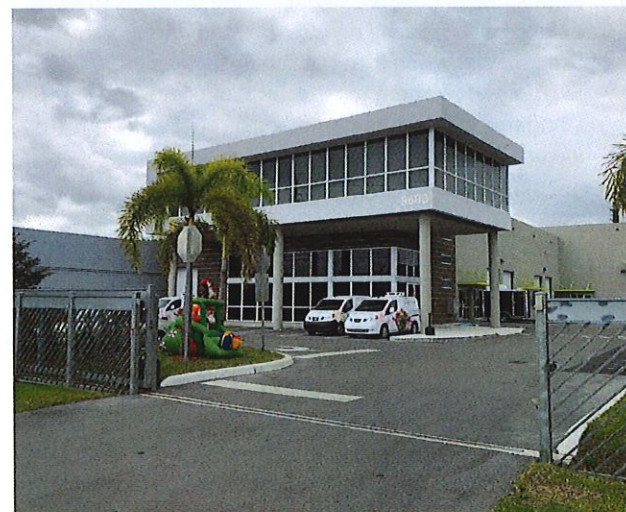
Figure 2-8: Example of Recent Development
