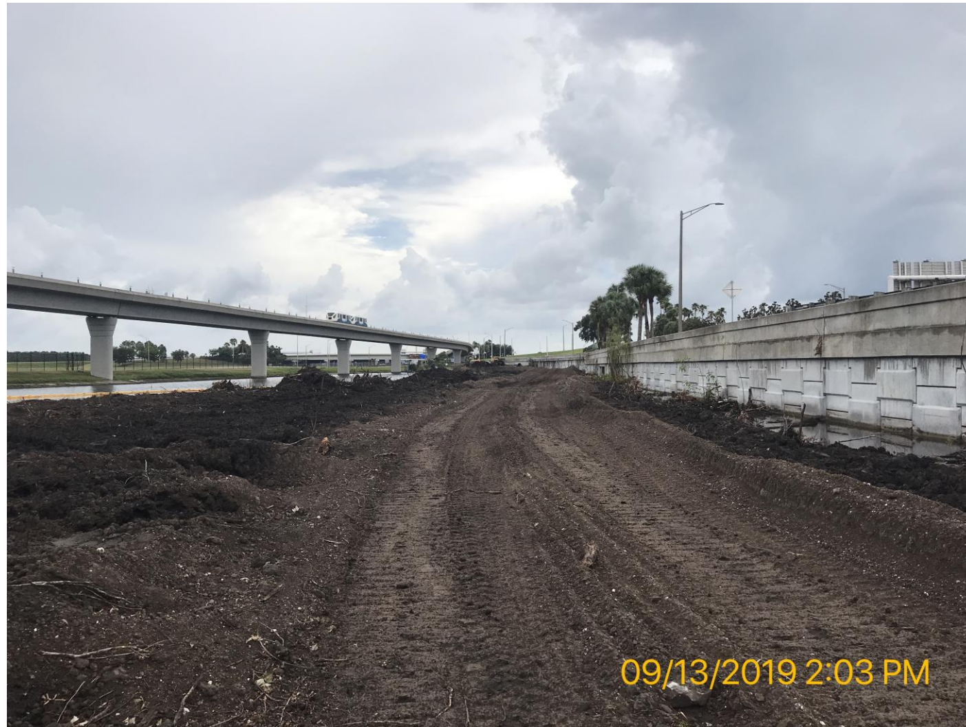
Clearing and Grubbing
