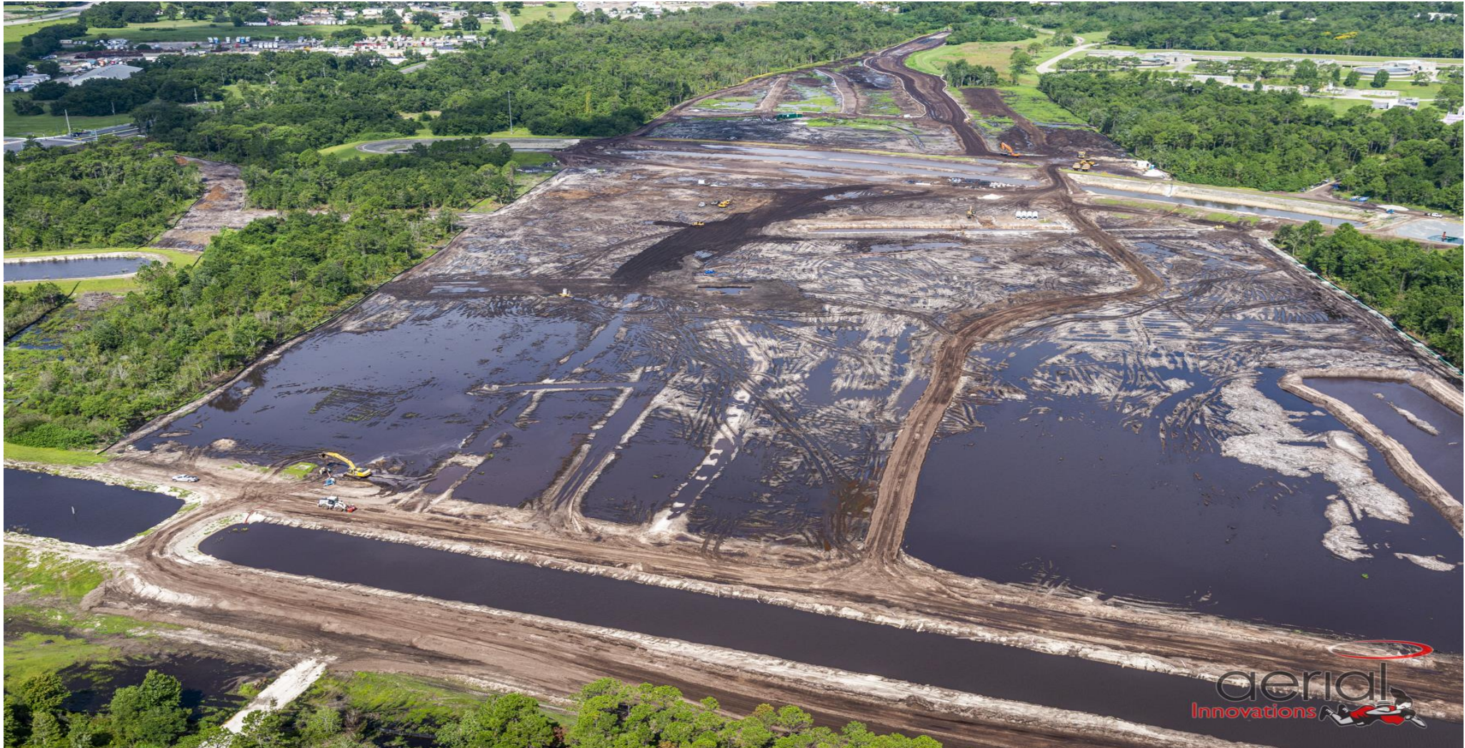
Clearing at the Vehicle Maintenance Facility
