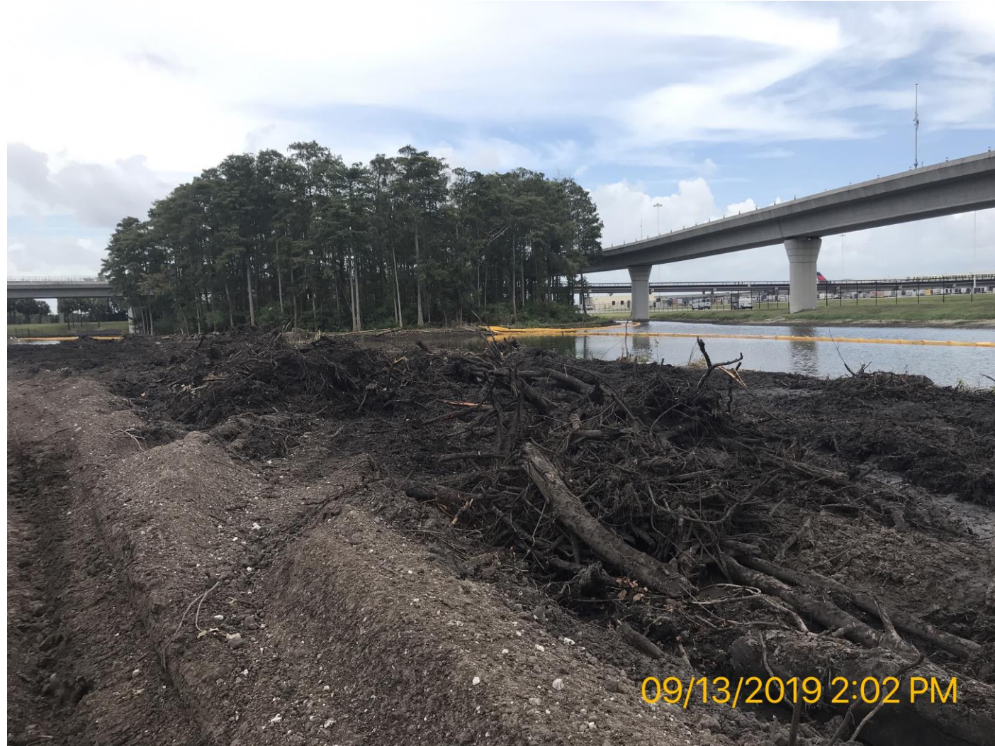
Clearing and Grubbing
