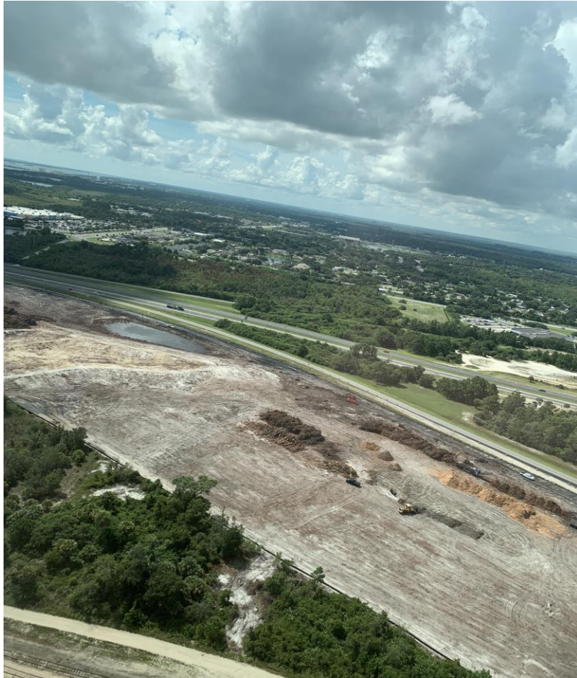
Clearing at Route 1
