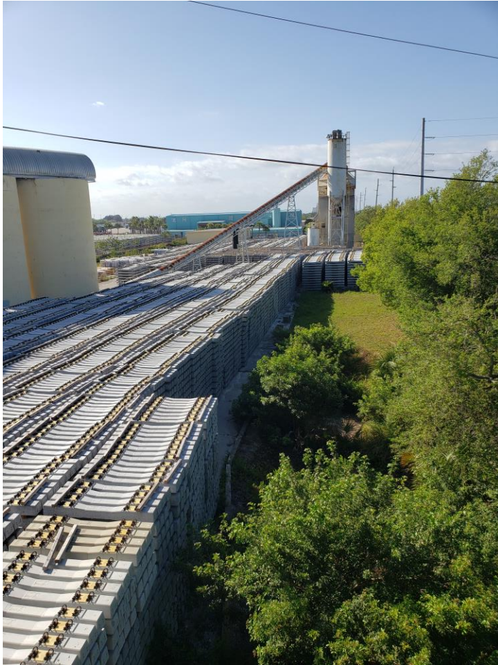
Rail Ties Delivery
