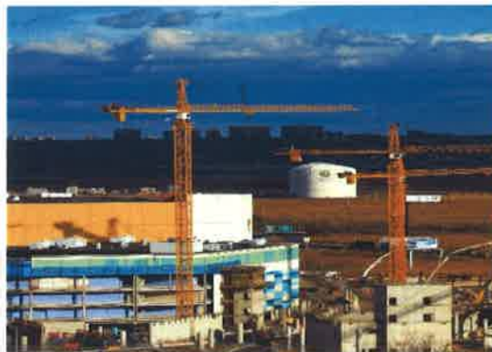
The American Dream construction site in New Jersey.
