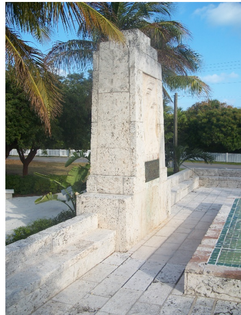
The Hurricane Monument in Islamorada
